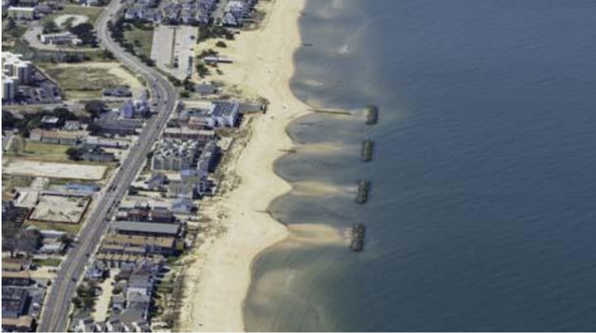
Figure 10-22. Breakwaters as erosion control (courtesy Virginia Institute of Marine Sciences).
