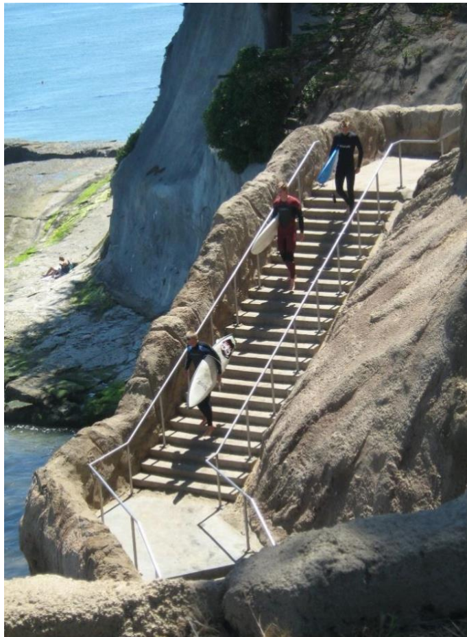
Figure 10-16. East Cliff Soil Nail Tie-Back Wall with Stairs for Coastal Access. Source: Surfrider Foundation.
