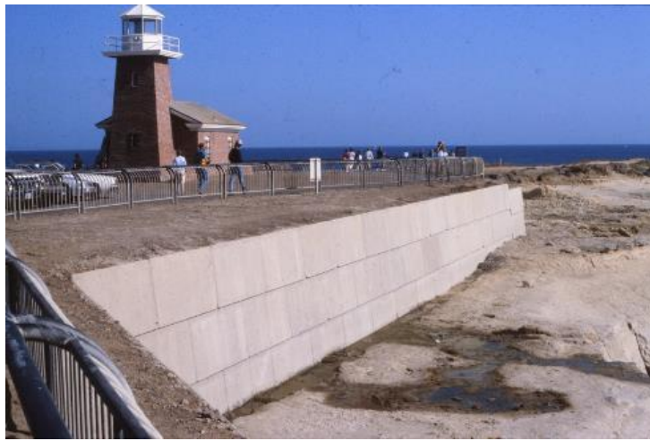
Figure 10-14. Upper bluff stabilization seawall at Lighthouse.
