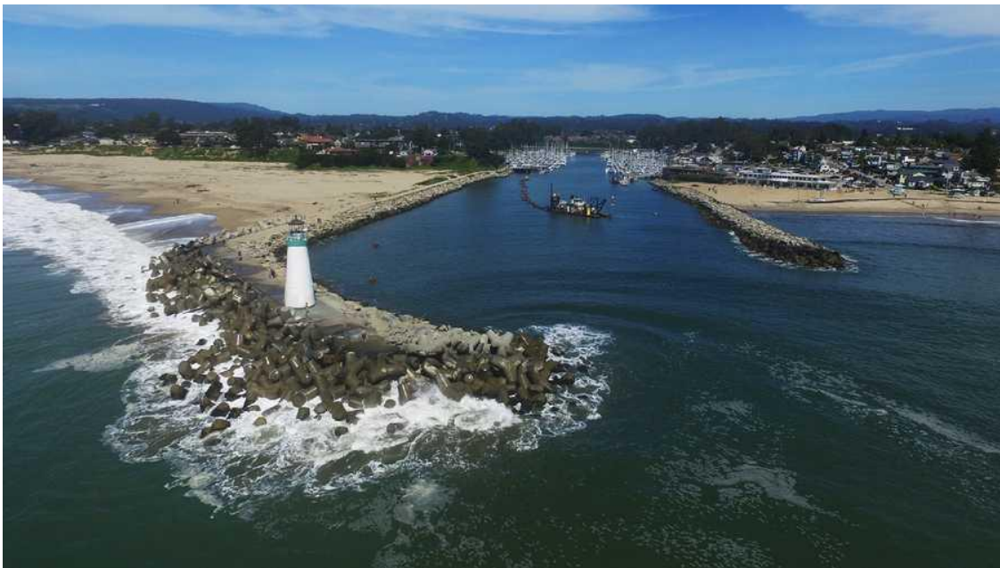
Figure 10-20. Santa Cruz Harbor Jetty retaining sand upcoast (to the left) on Seabright State Beach. Source: KSBW, Steven Morgan.
