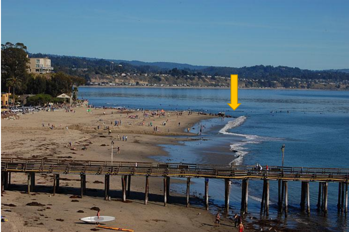
Figure 10-21. Capitola Village groin (in yellow) showing the widened recreational beach that also helps to reduce wave impacts.
