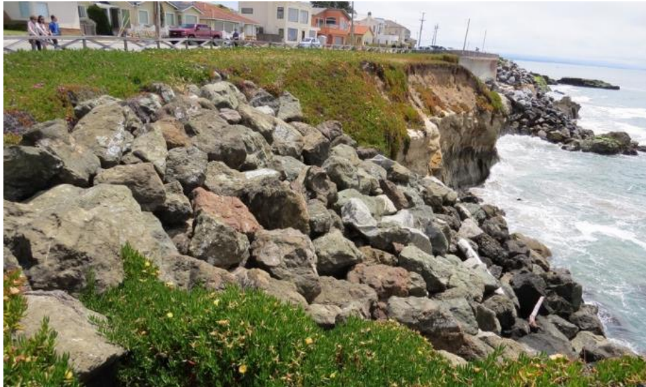
Figure 10-13. Revetment along West Cliff Drive near David Way in Zone 2.
