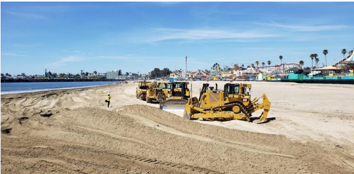
Figure 10-27. Sand management at the San Lorenzo River Lagoon addresses beach changes to lagoon opening and closing caused by the Santa Cruz Harbor sand retention.
