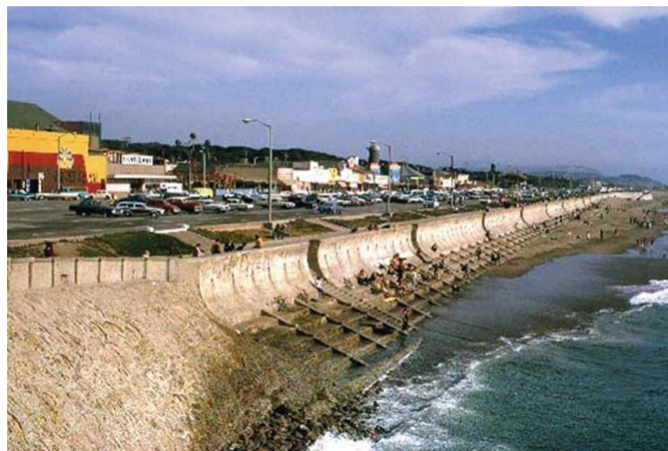
Figure 10-15. Recurved seawall in San Francisco designed to reduce wave reflection and support sand accumulation.
