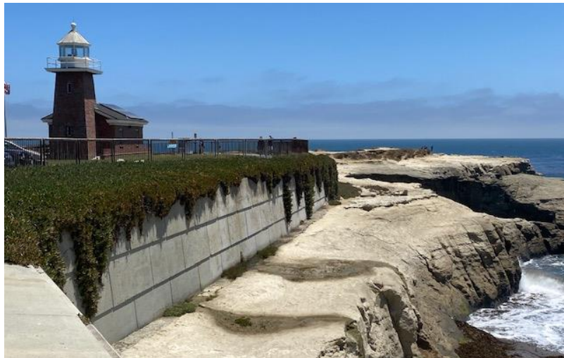
Figure 50. Bluff top seawall at Lighthouse Point
