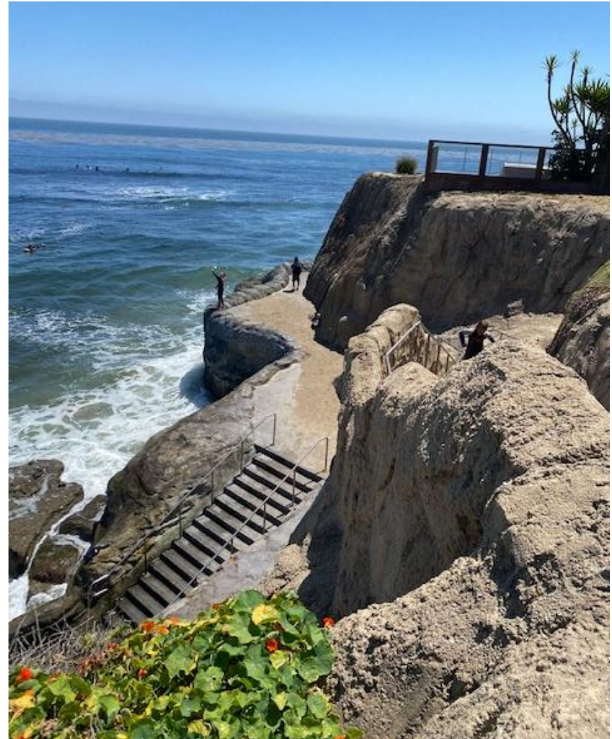
Figure 51. Soil nail wall with vertical beach/ocean access stair at Pleasure Point
