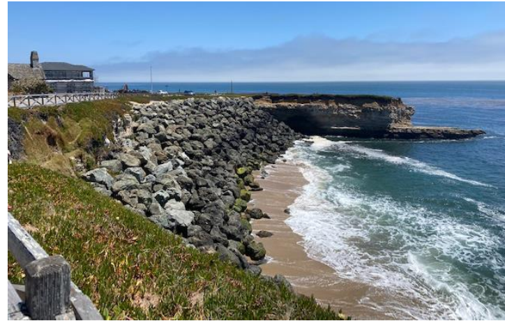
Figure 9. Rip rap backs many of the West Cliff pocket beaches
