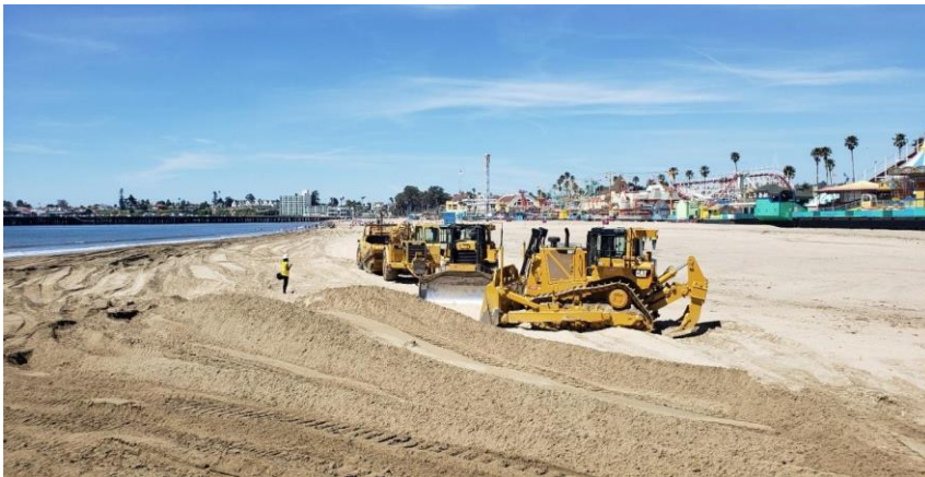
Figure 58. Beach contour management along Main Beach by the San Lorenzo River mouth
