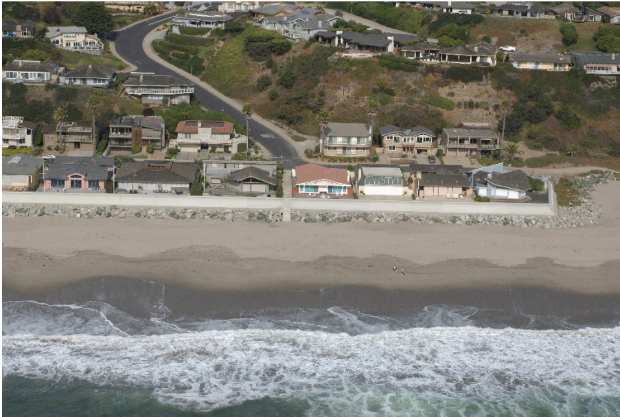
Figure 1: Example of Seawall in Aptos, Santa Cruz, California Coastal Records Project. Copyright © 2008 Kenneth & Gabrielle Adelman. All rights reserved.
