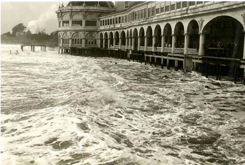
Figure 12. Severe storm went through Santa Cruz, causing flooding. February 13, 1926. Source: SF Chronicle
