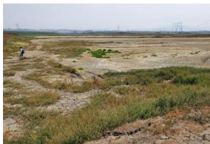
(B) 2020-initial earthmoving complete
