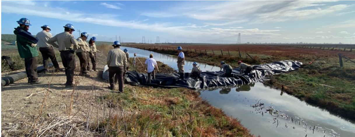
Figure 8. California Conservation Corps crew working with CCWG on the construction of the Moro Cojo Slough weir.
