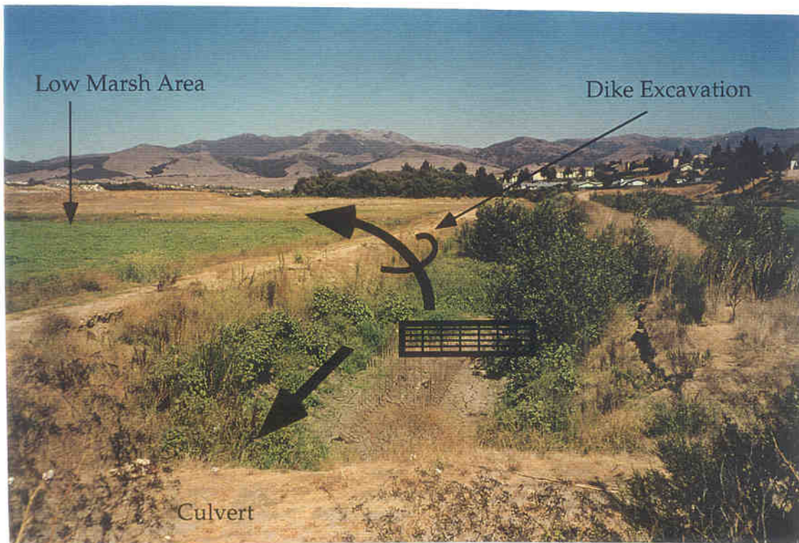
Photograph 8. Ponding also permits water to enter the low marsh next to Laurel Lake through a low area excavated in the ditch dike. Thick arrows indicate water flow.
