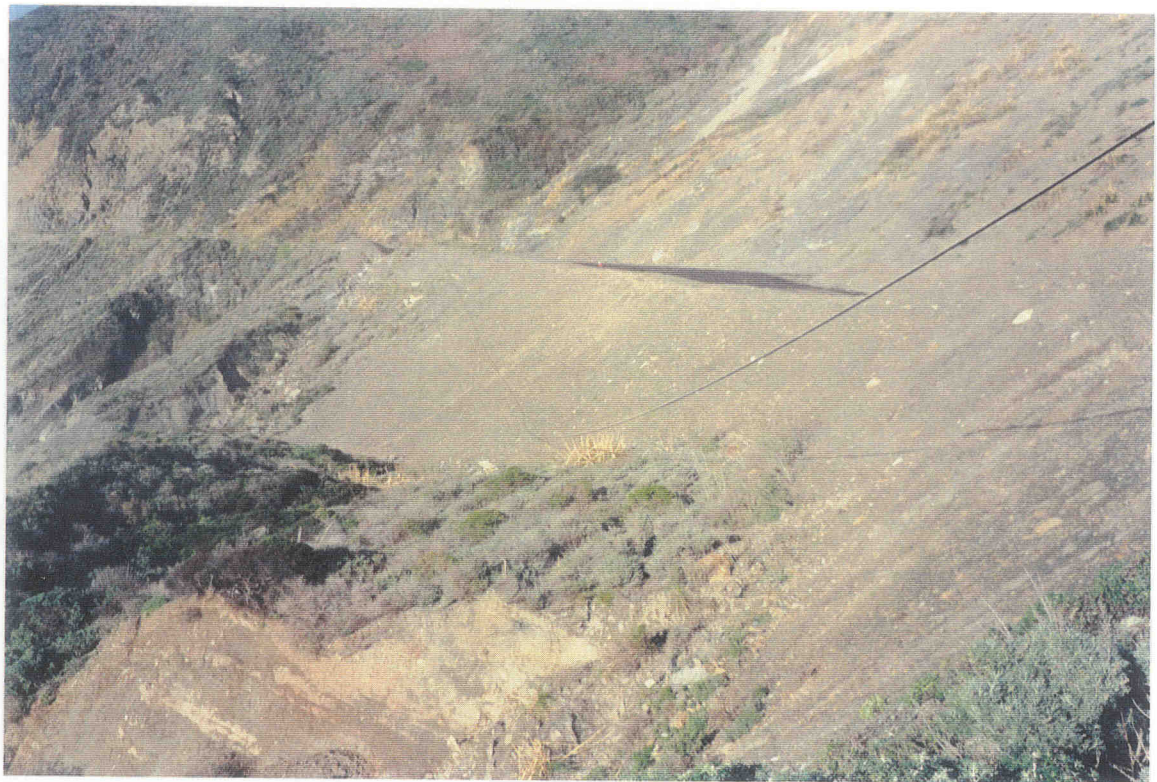
Figure 11. Two more creeping landslide along the Big Sur coast which are deposition sites for landslide debris on the highway.
