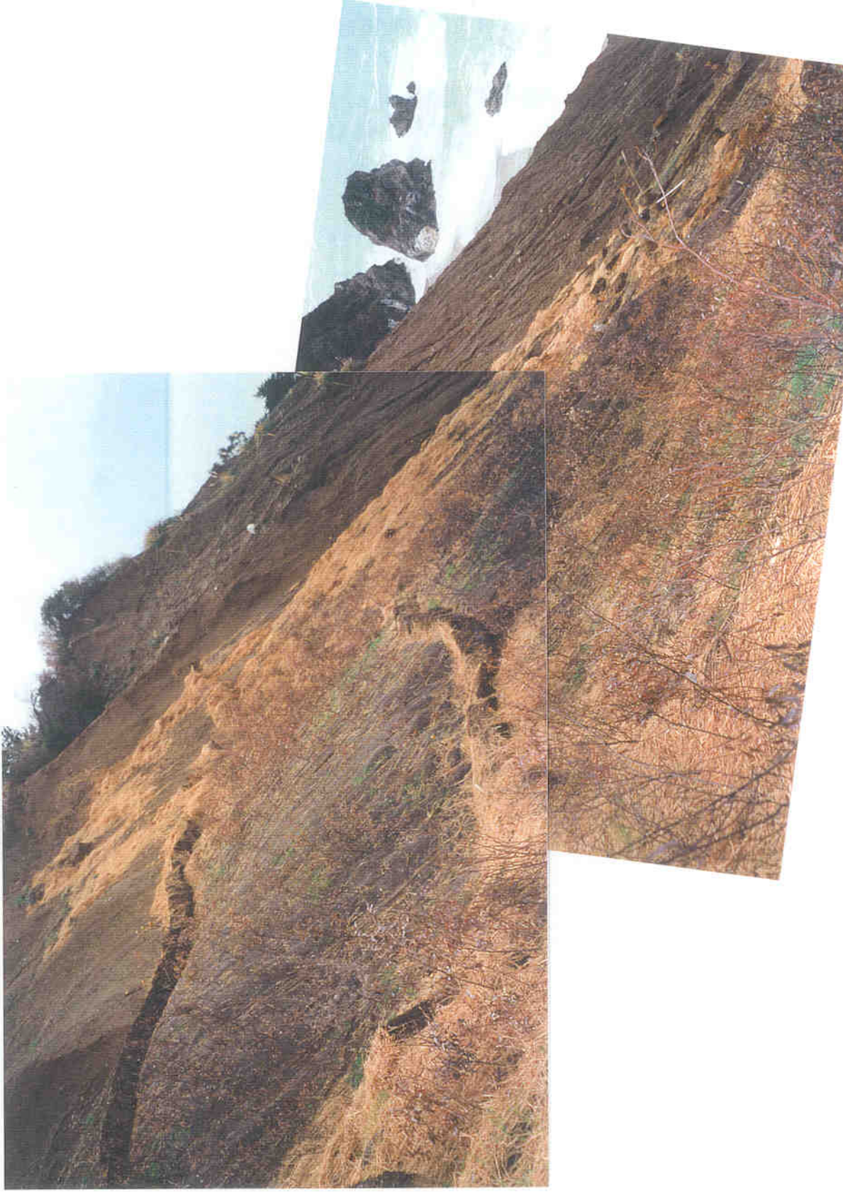
McWay landslide on January 4, 1998 after some rain damage, willow cuttings plugged 3-4 feet apart hay, seed, and nutrients spread over exposed soil.
