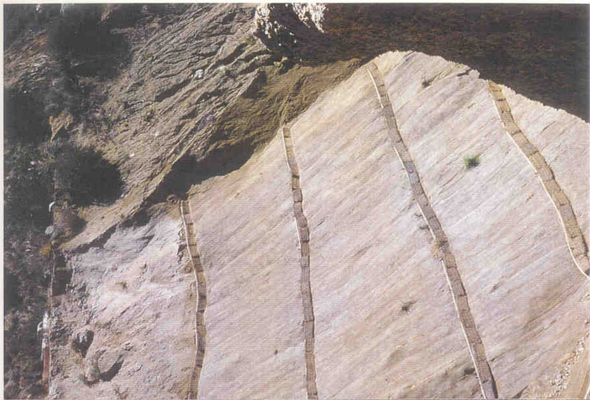
McWay Landslide in October 1997 Seed, Hay, Jute, Haybales and Irrigation (no nutrients)
