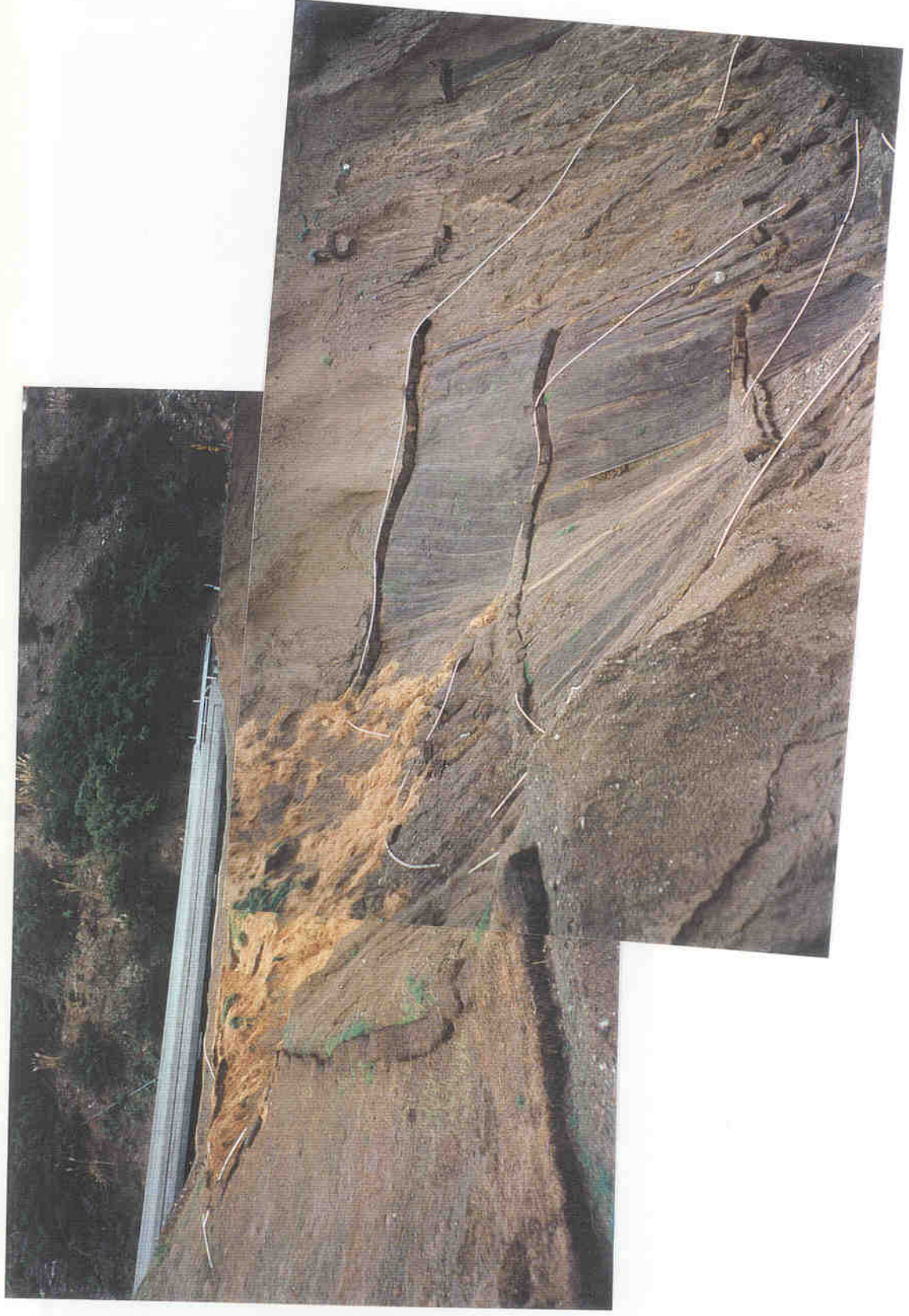
McWay landslide on December 9, 1997 after two major rains (1 and 2 inches), jute slumped from southern portion, surviving irrigation, first hay, seed, and nutrient treatment just beginning in the bowl.
