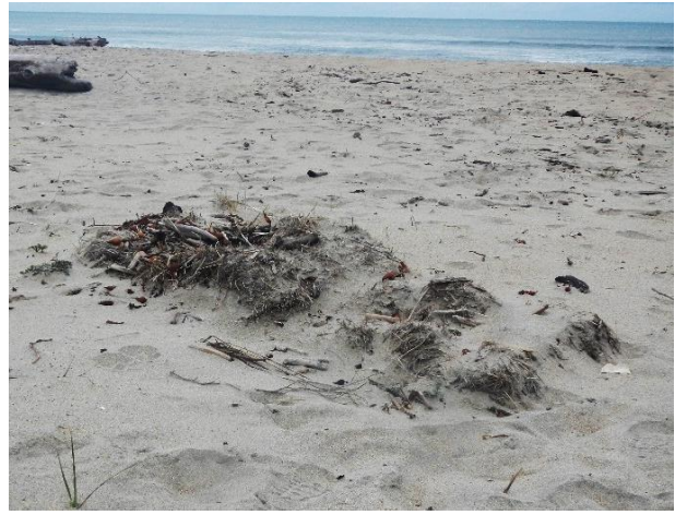
Figure 4. Installation of drift wood and hay bales along the foredune help capture sand and increase dune roughness. Left: Initial placement of hay bales and driftwood near the Potrero Rd beach access trail. Right: After a few months the hay bales slowly decompose while continuing to help capture sand and add to foredune roughness.
