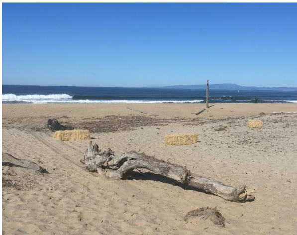
Figure 4. Installation of drift wood and hay bales along the foredune help capture sand and increase dune roughness. Left: Initial placement of hay bales and driftwood near the Potrero Rd beach access trail. Right: After a few months the hay bales slowly decompose while continuing to help capture sand and add to foredune roughness.
