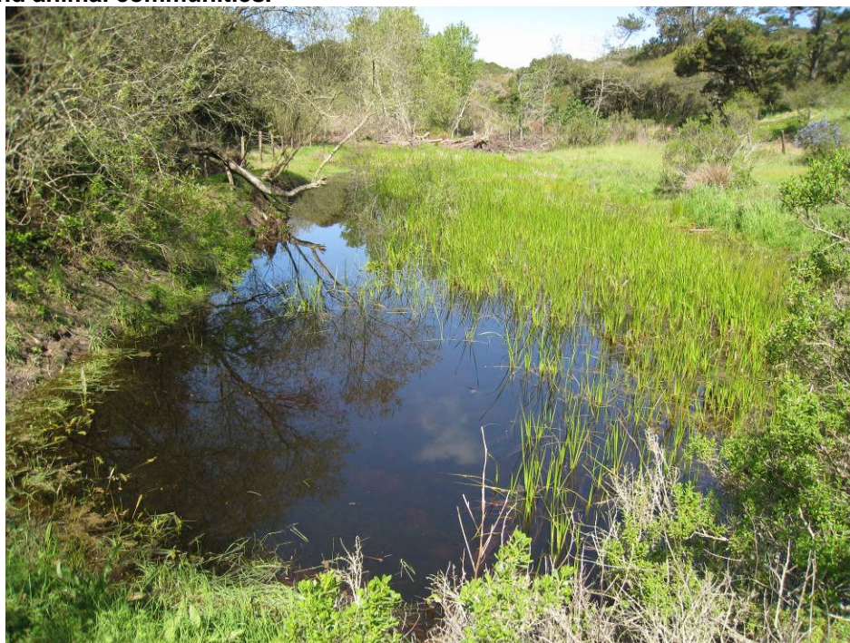
Figure 19 The downstream end of Wagner pond in March 2008. Several BMPs are illustrated by the reduced soil erosion and flooding and the improved pond hydrology resulting from the new culvert installation, as well as by the positive impacts on wetland plant and animal communities.
