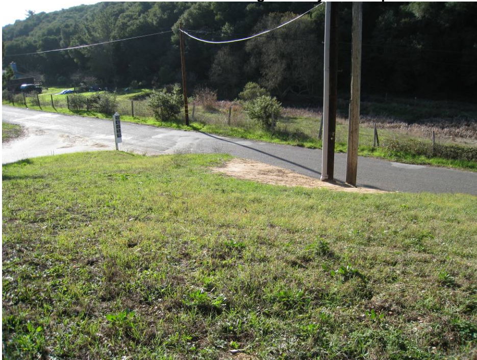
Figure 15 Looking from the water capture basin towards Wagner pond. We extended the culvert from the road's edge directly into the pond
