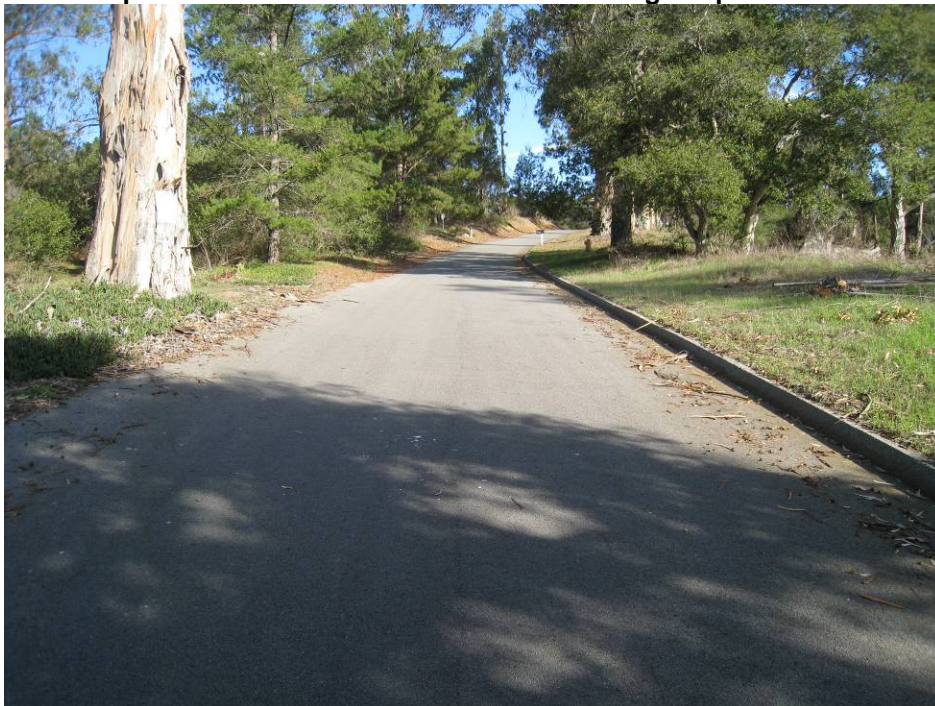
Figure 12 The watershed above the Wagner property is dominated by a wide road and at least as much impervious surfaces at each home site along the private road.
