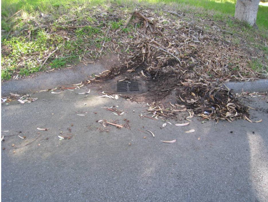
Figure 13 Water running down the road is captured in this drain and sent to a holding pond.
