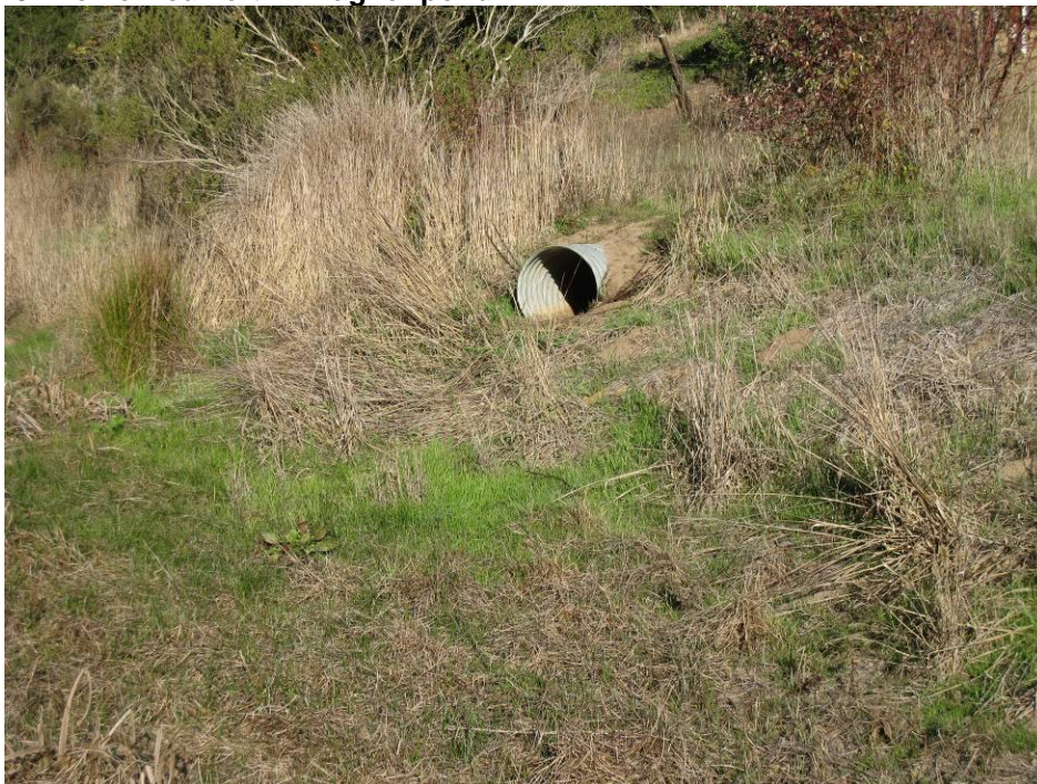
Figure 16 The new culvert in Wagner pond
