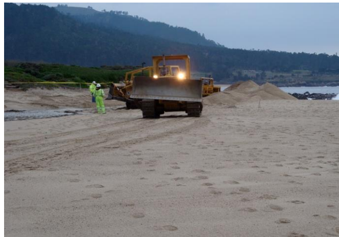
Figure 4.2: Active beach berm management at Carmel River mouth
