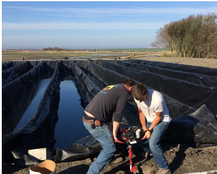
CCWG STAFF BUILDING THE MULTI-CHAMBER BIOREACTOR
